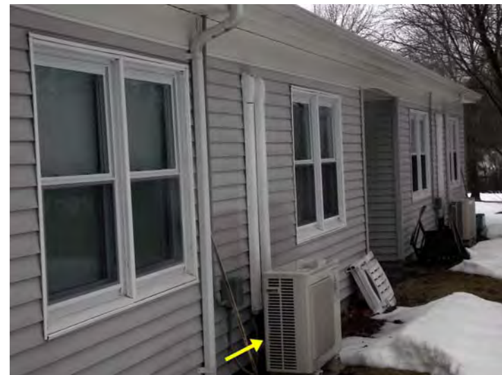
This is the heat pump condenser unit.
