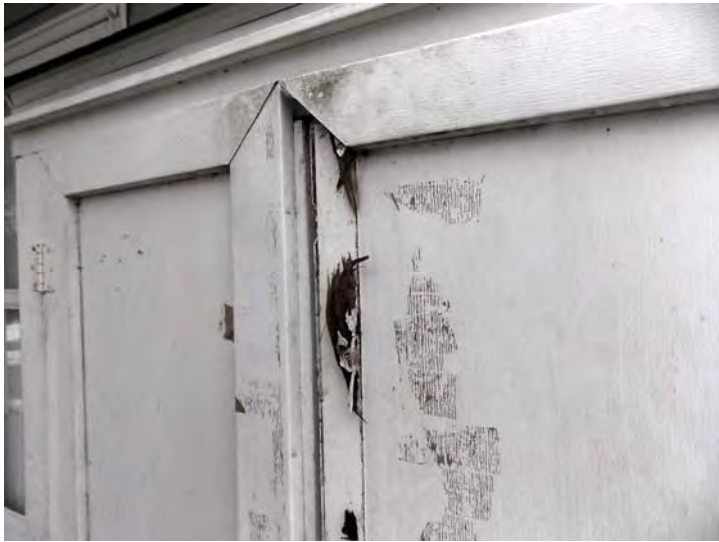
A close-up of a deteriorating wood door frame.
