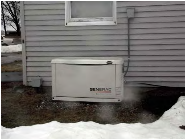
This is the emergency generator; it provides 10 kW of power to the community building.
