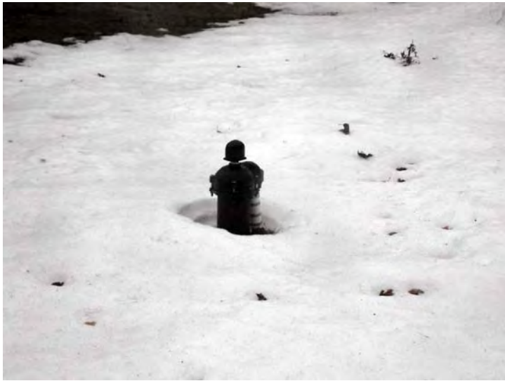
This is the well-head for the domestic water well.
