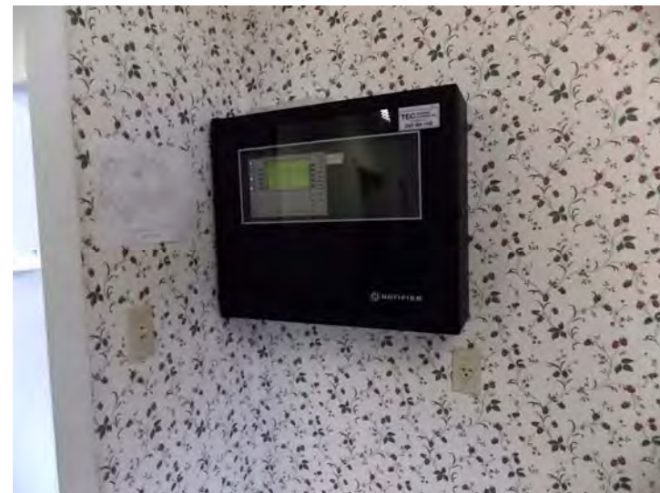
The central fire alarm control panel.
