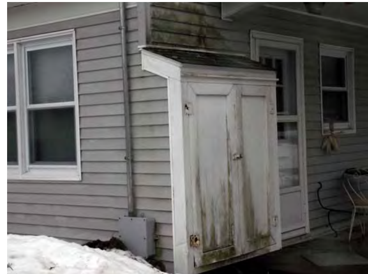
Moisture-related vegetation growth on a wall section and storage door.
