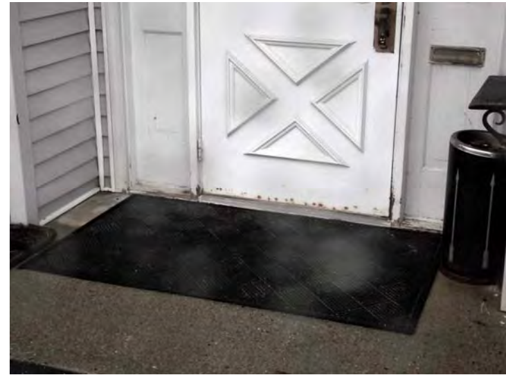
Note the rust at the bottom of the door (Community Building).
