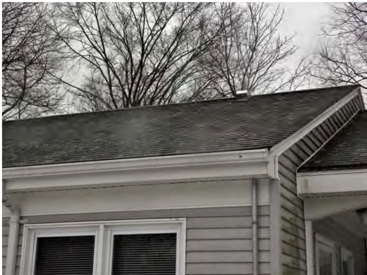
Roofs are covered with asphalt shingles and have gutters and downspouts.
